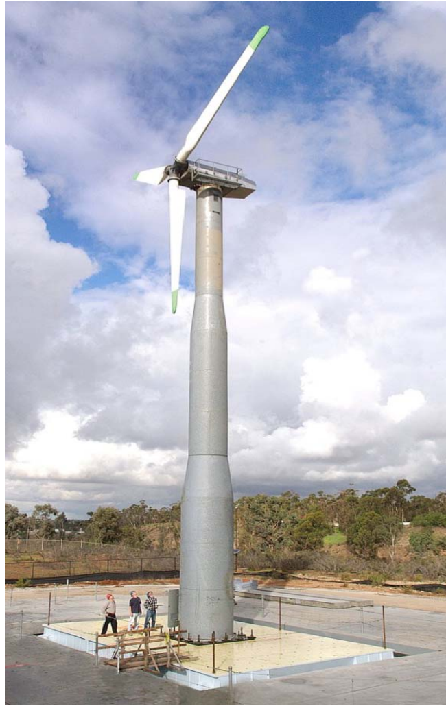
Figure 4 – 22.6m Hub Height Turbine Mounted on UCSD/NEES Shake Table [from Prowell, Veletzos, Elgamal, 2008]
